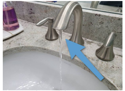
Master Bathroom left sink
